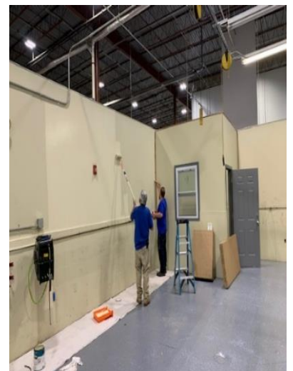
New office space in the mechanic shop at 2900BCD.
