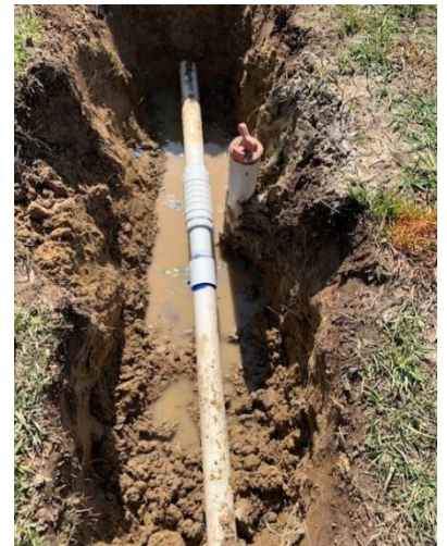
Irrigation repair at Founders Park.
