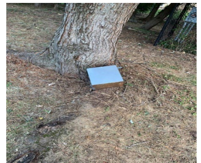
Electrical box/wires secured at Fort Ward Park after.
