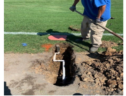
Boothe Softball/Irrigation after
