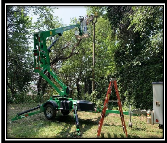
These photos are at Ewald Playground. We converted the old existing metal halide lights to LED
