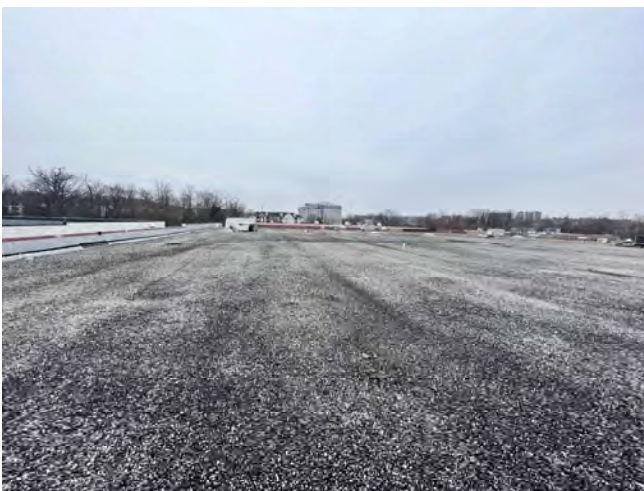
23. Built-up roof topped with pea gravel
