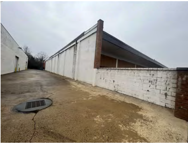
3. Left (south) elevation of building
