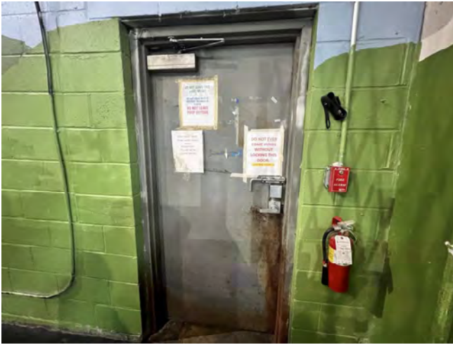
19. Interior of exterior door
