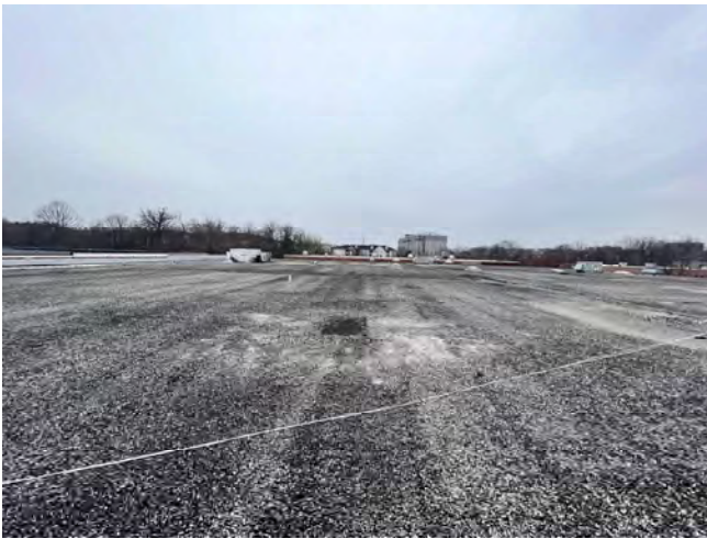
21. Built-up roof topped with pea gravel
