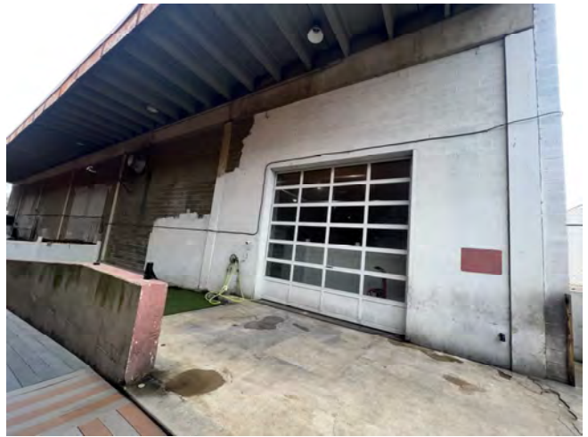
4. Rear (west) elevation of building
