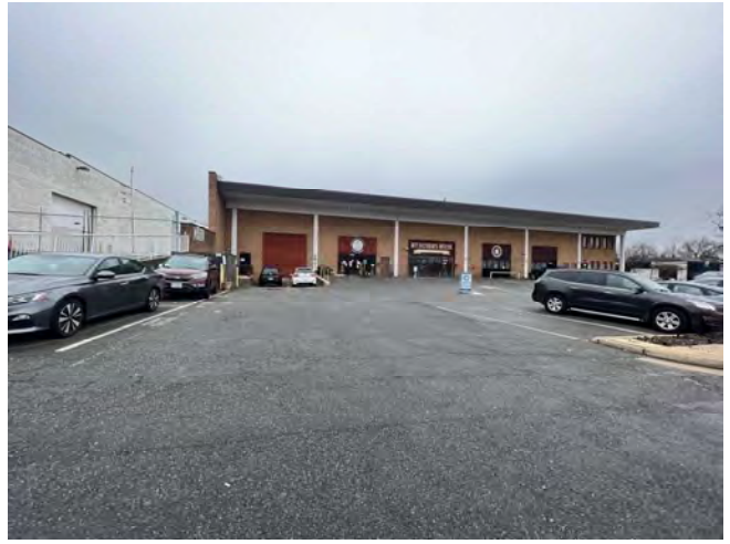
2. Front (east) elevation of building
