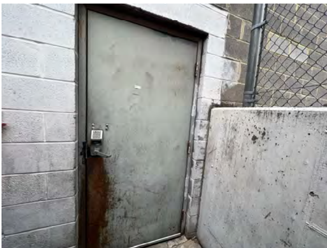
17. Exterior of exterior door
