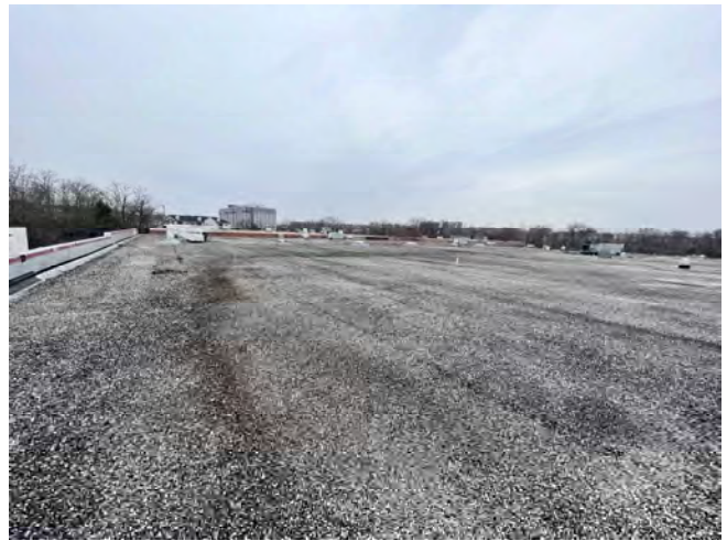
22. Built-up roof topped with pea gravel
