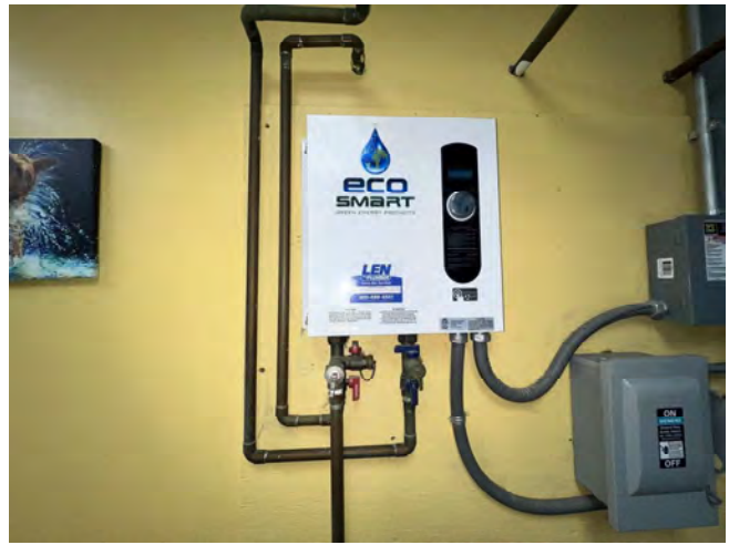
26. Instantaneous hot water heater
