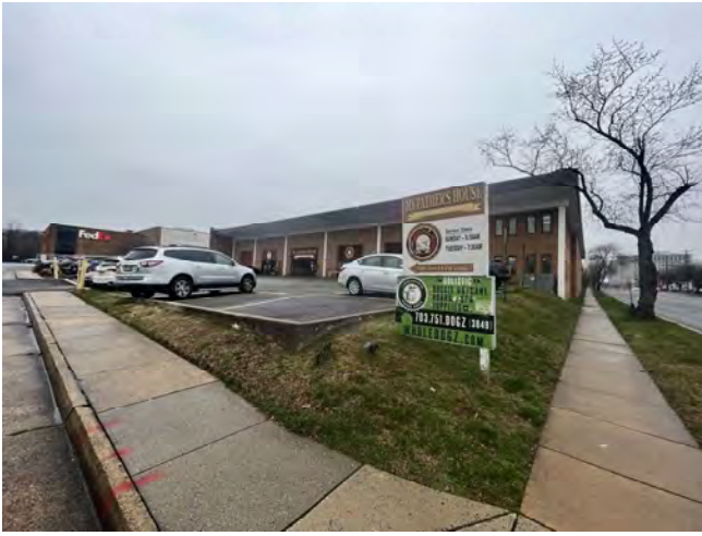
1. Street view of Subject Property
