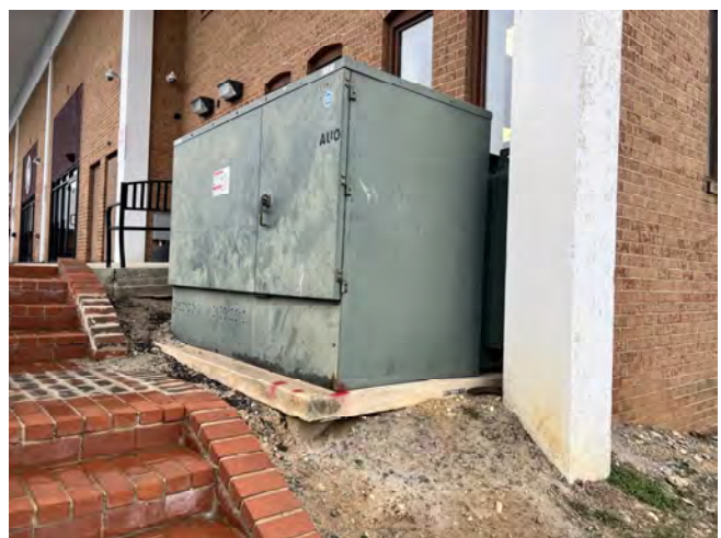
30. Pad-mounted transformer
