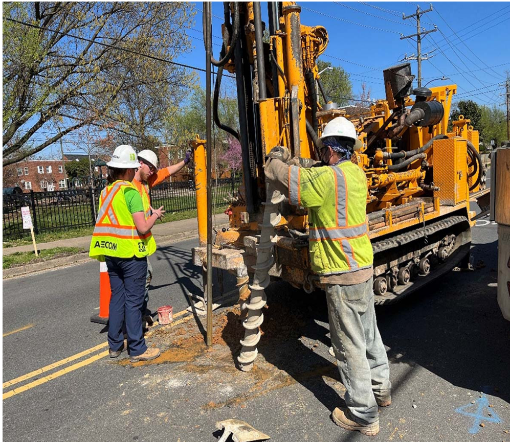
Watch a video of crews at work on W. Reed Ave.
