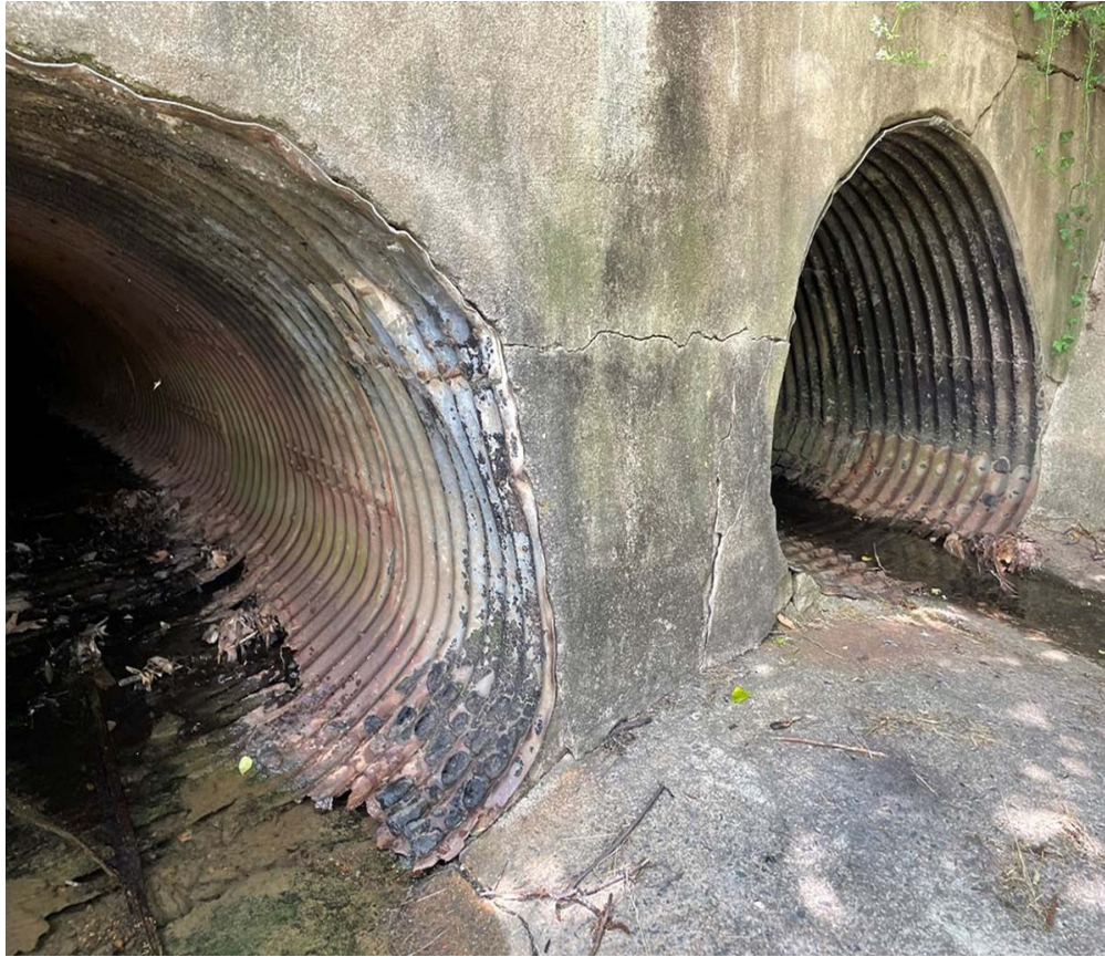
Dual culverts at headwall
